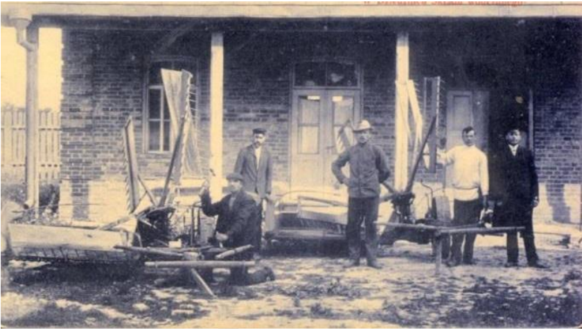
Wine processing plant, mechanical workshop, early 20th century
