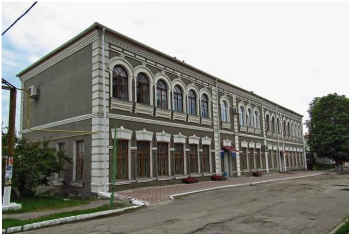
The former trading house of the 1 st guild merchant, B. Ya. Kats. Built late 19th century.
