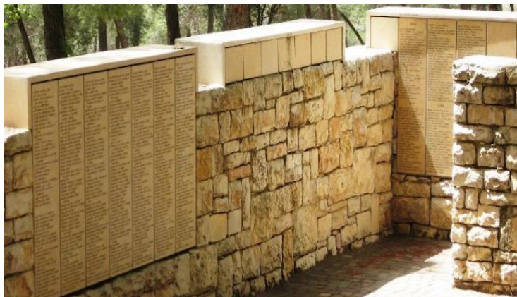
Memorial wall in the Garden of the Righteous with the immortalized names of the Righteous and their country of residence
