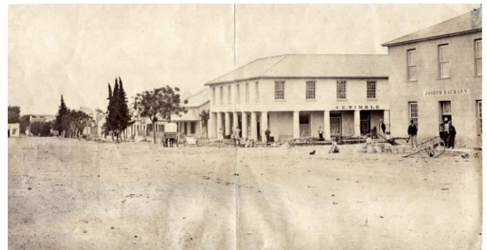
The Joseph Baumann building in Graaff-Reinet, later taken over and renamed Wille & Wertheim
