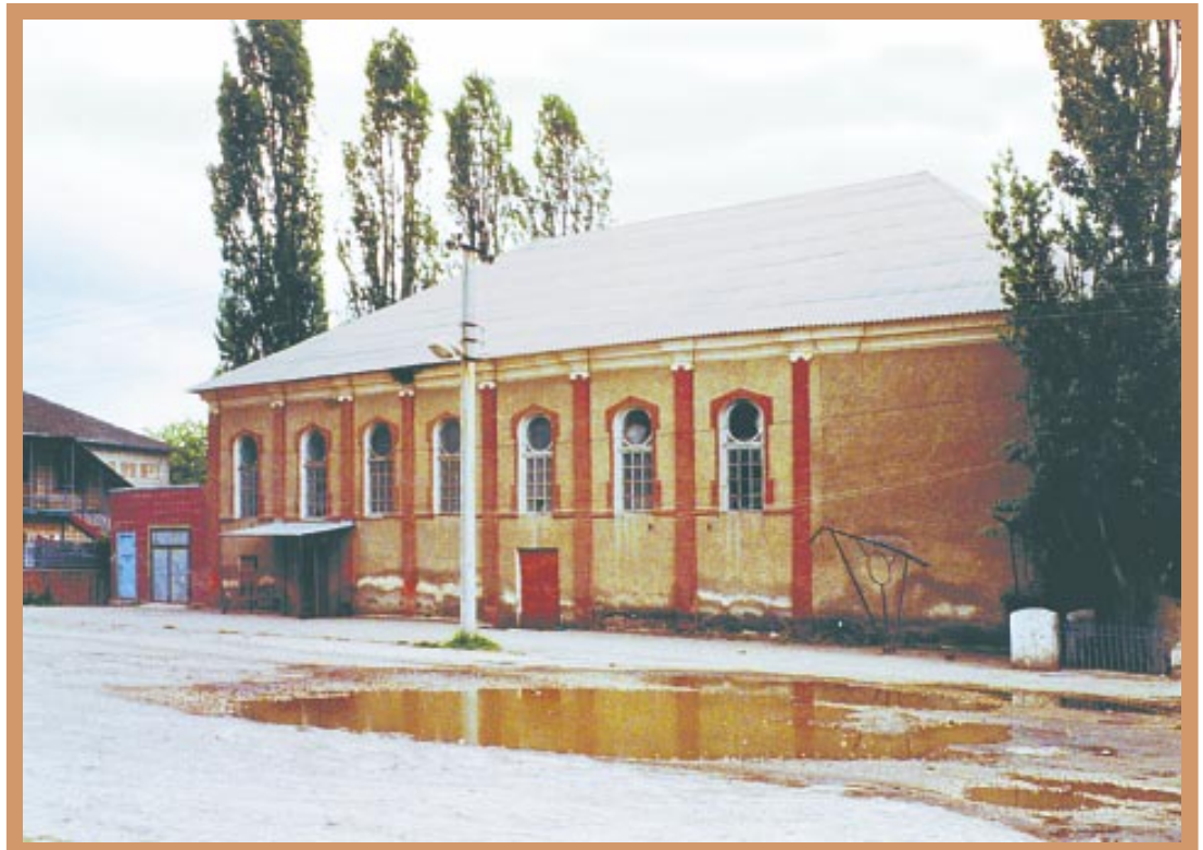
■ Former synagogue in Ataki, now a cultural center, 1992
